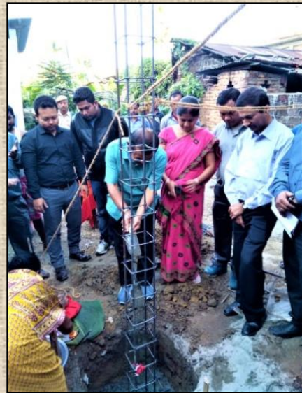
Laying of foundation by Ward Councillor on 19/01/2018, Dibrugarh Municipal Board
